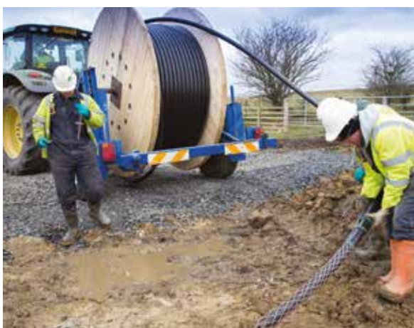
7. Pull cables into ducts
