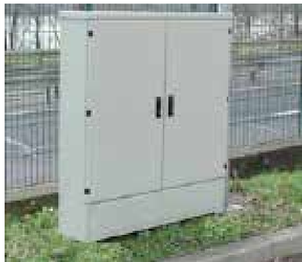
Cable corridor post reinstatement, with link box at field boundary
