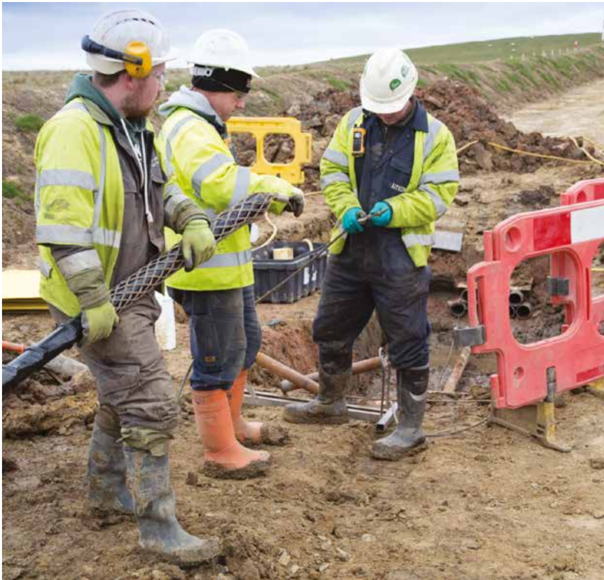
Cable pulling preparation
