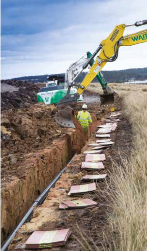
3. Ducts Covered and Protective Marker Tiles Laid
