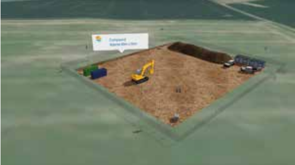
1. Site establishment including topsoil strip and store
