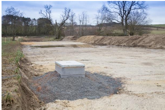
Cable easement prior to reinstatement, with link box.
