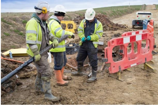
Attaching the pull-wire to the pulling sock
