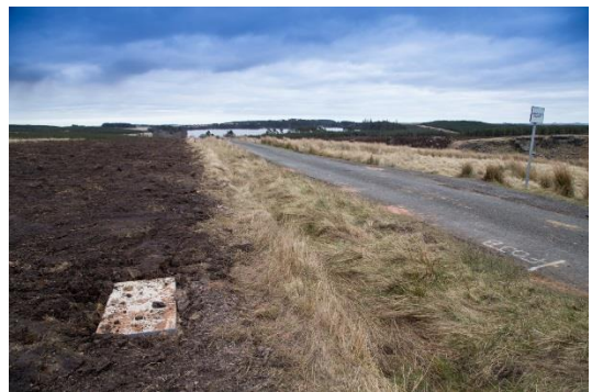
Cable easement after reinstatement, with link box in foreground.
