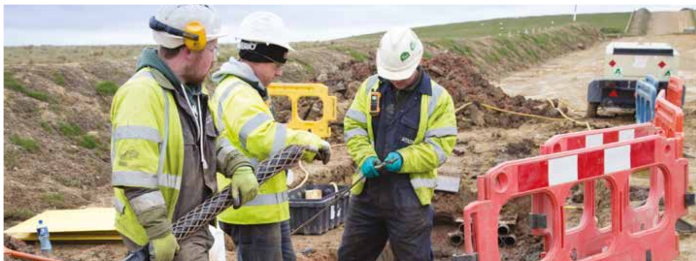
Cable pulling preparation
