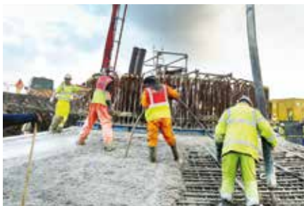
Over 400 cubic metres of concrete and 2 days using large concrete pumps.
