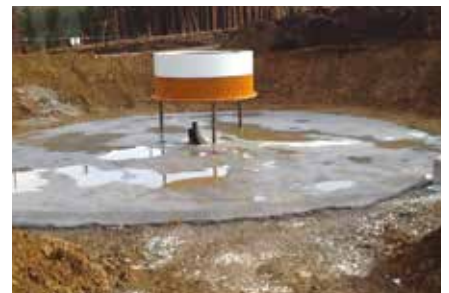
A layer of stone and concrete to create a clean working area.
