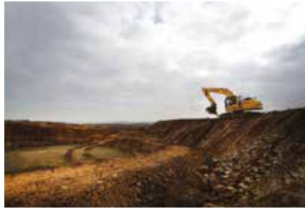
Turbine foundation excavations, approximately 20m diameter, 3m deep.
