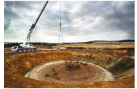
2 men 6 days to piece the steel reinforcement together.
