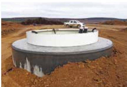
Backfilling of each foundation completed leaving the upstand exposed for the turbines to be bolted onto.
