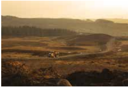
11.2km of site roads.
